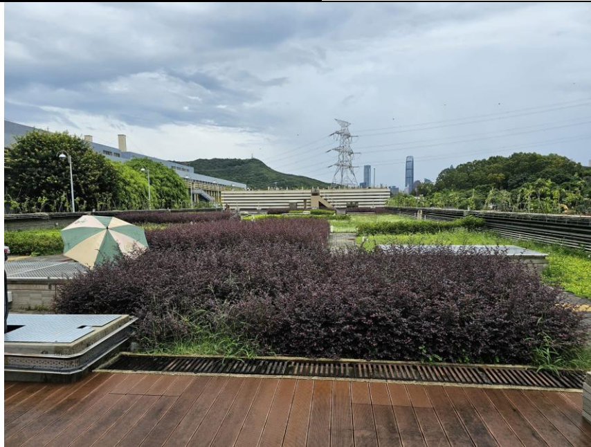
General view of HCF Roof Landscape Softworks
