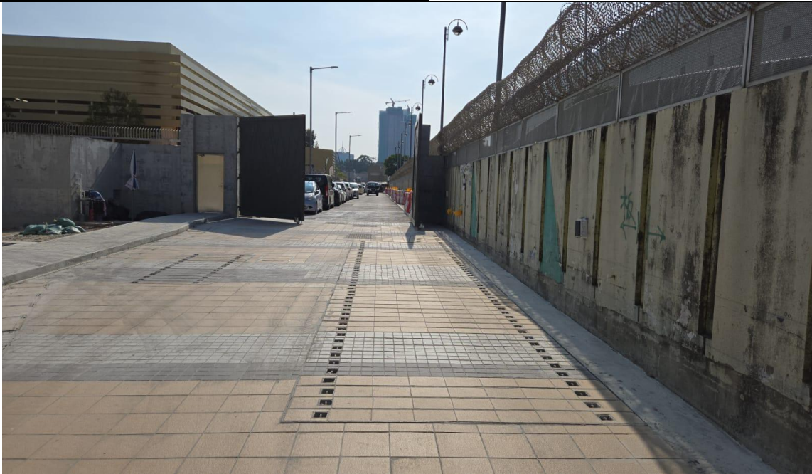
EVA Tile Paving Work
