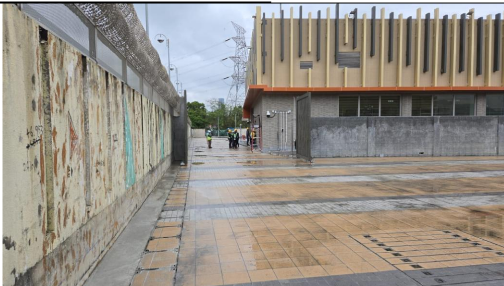
Gate 1 and Gate 2 Modification Works
