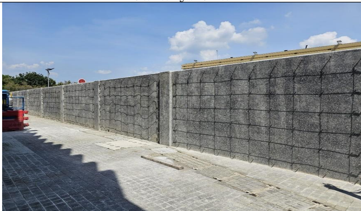
Installation of Vertical Green Mesh
