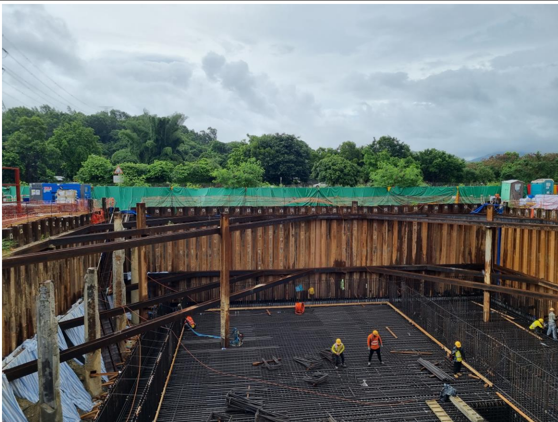
Rebar fixing work for Reclaimed Water Pumping Station
