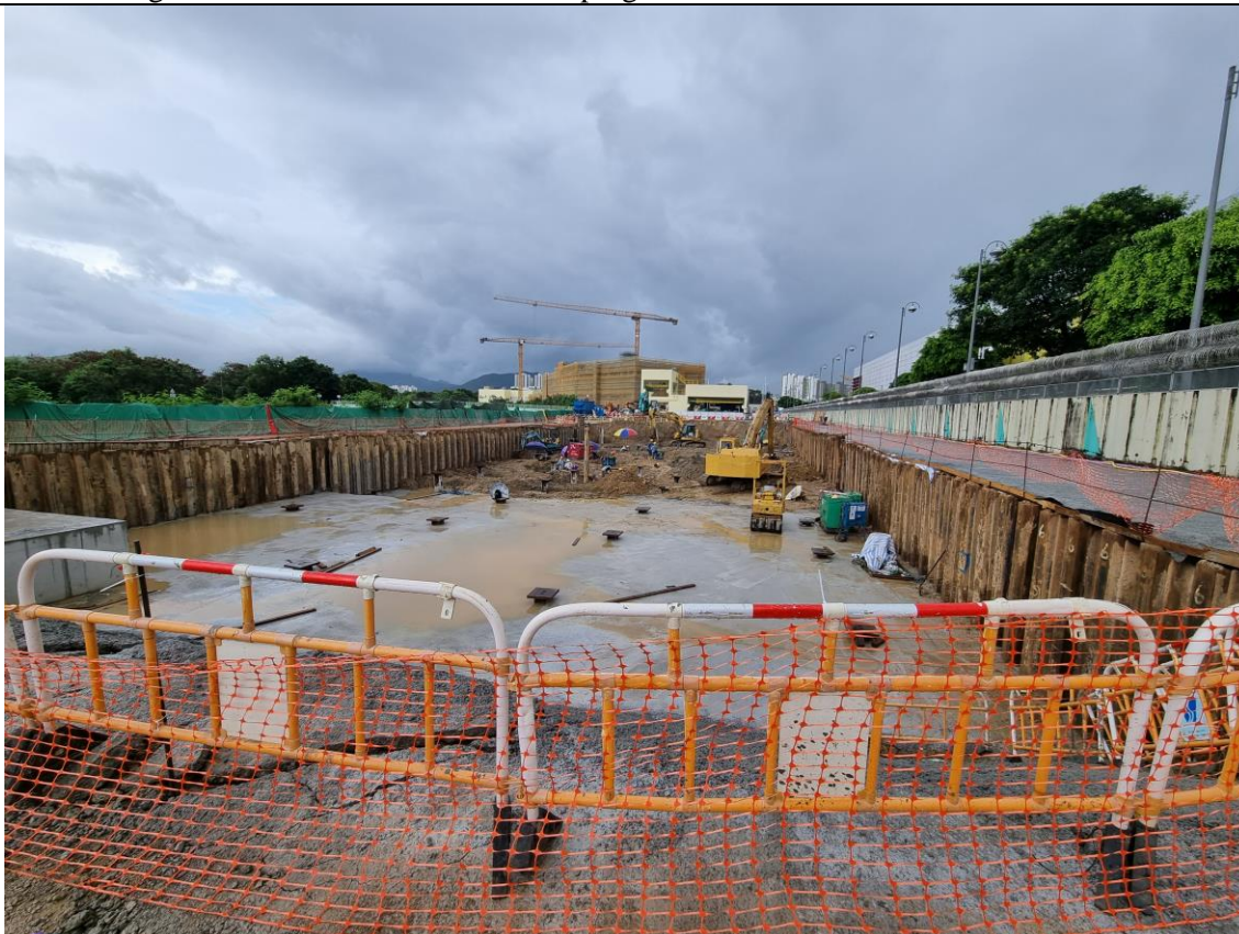
Excavation and lateral support work for Hypo-Chlorination Facilities
