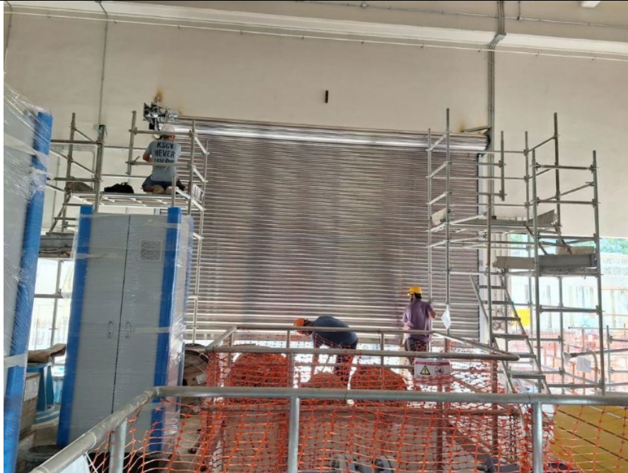
Metal works at HCF
