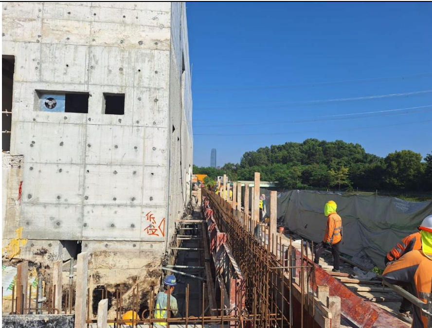
External Works at SWHWP
