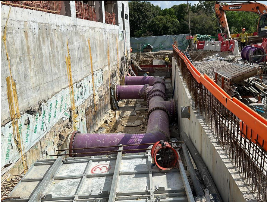
External Works at SWHWP
