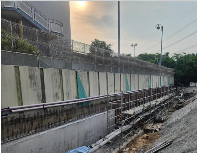
Fence wall at SWHWRP – Rebar fixing and Concreting work
