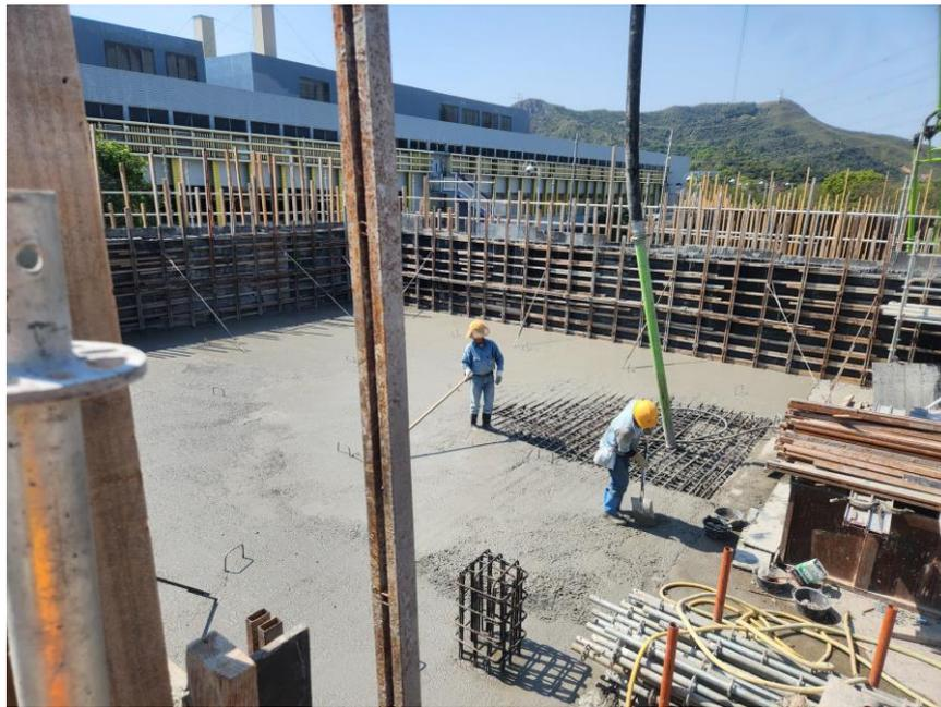
R.C. Structure of HCF - Concreting work at Roof Floor
