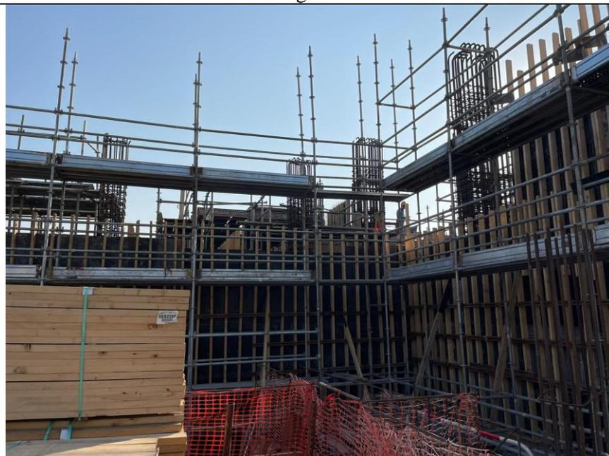
R.C. Structure of ReWPS - Formwork Erection and rebar fixing work for Wall & Column up to Corbel
