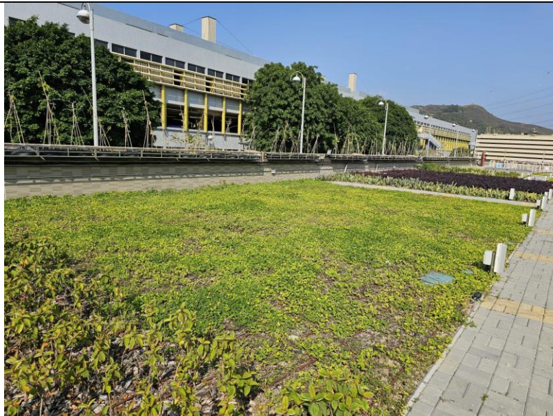
General view of HCF Roof Landscape Softworks
