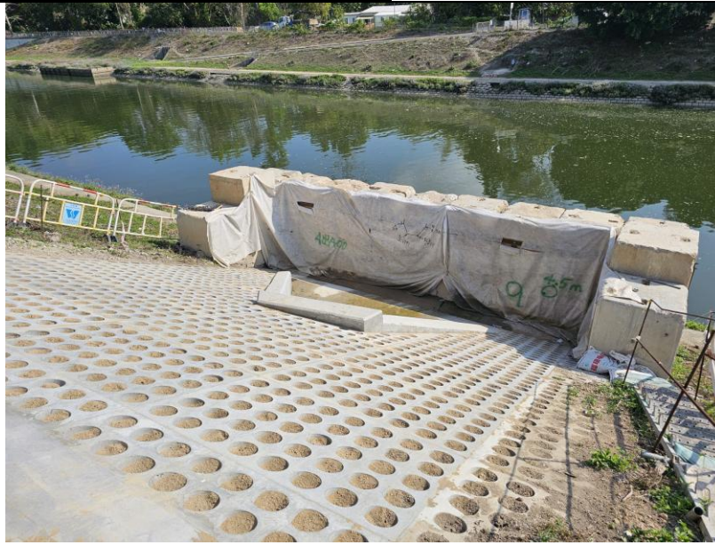
Construction of Outfall
