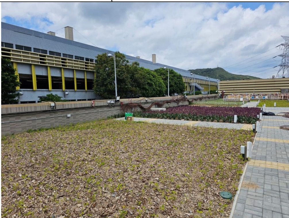
Landscape Softworks at HCF Roof
